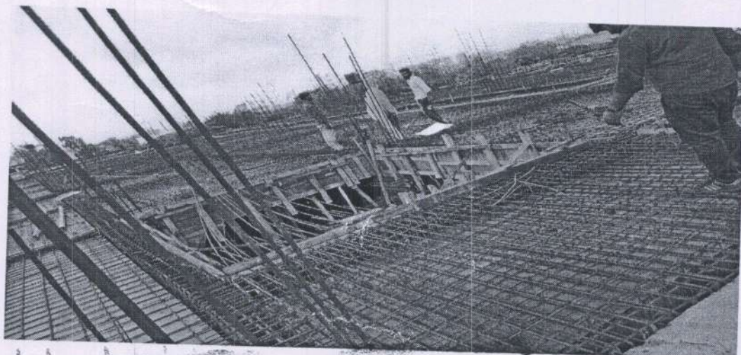
Fig 4: Footing reinforcement
