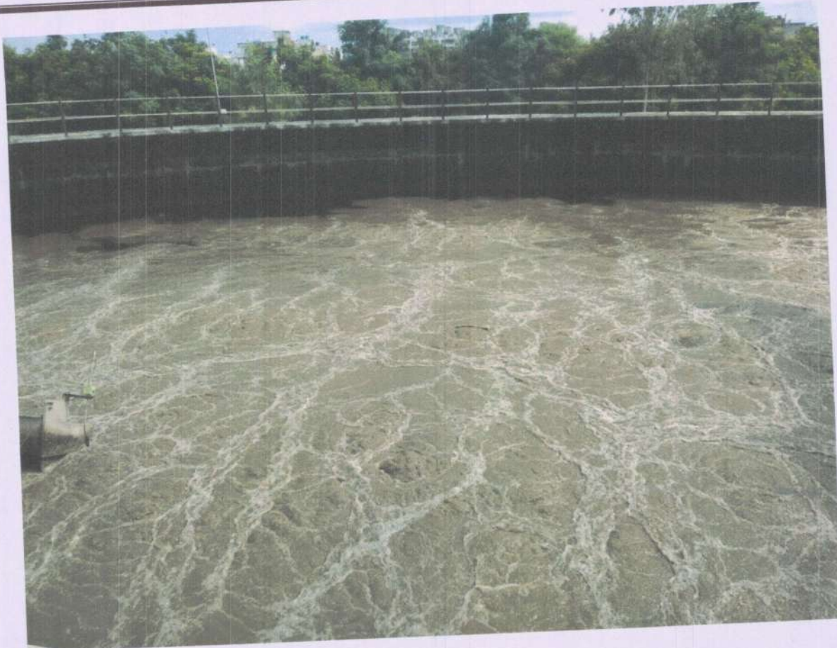
SBR BASIN : AERATION MODE
