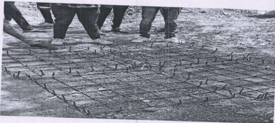
Fig 4: Footing reinforcement
